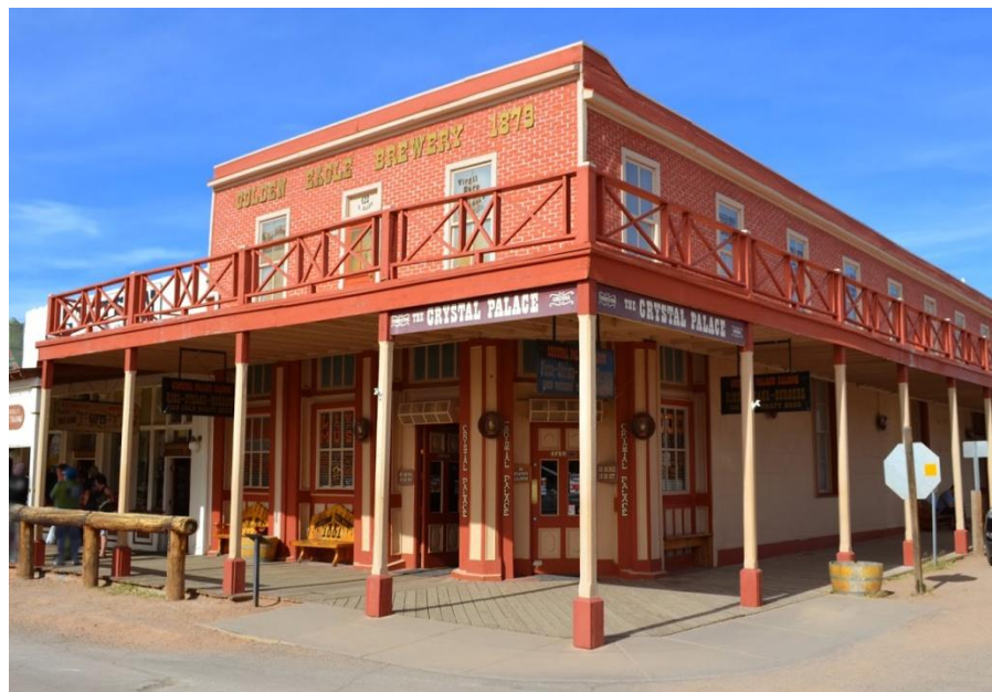
The Golden Eagle Brewery as it appears today following its meticulous restoration in the early 1960's. The Crystal Palace Saloon still operates on the ground floor.
